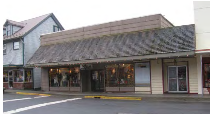
Figure 25. The Cellar at 200 Lincoln Street, view facing southwest (©TNSDS 2014).
