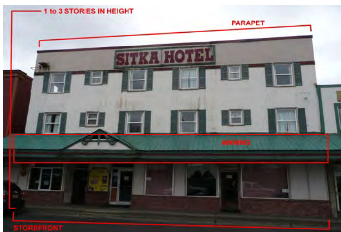
Figure 14. Example of a contributing building in the Sitka Historic Business District with primary features identified (©TNSDS 2014).
