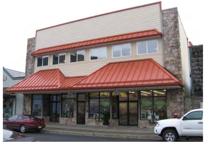
Figure 33. Troutte Center, 329 Lincoln Street, view facing southeast (©TNSDS 2014).
