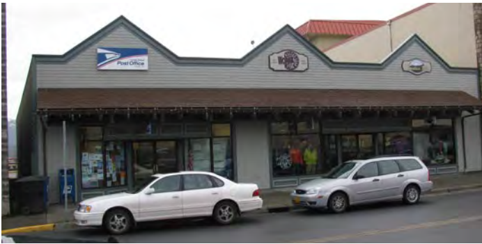
Figure 34. The U.S. Post Office at 334 Lincoln Street, view facing southwest (©TNSDS 2014).
