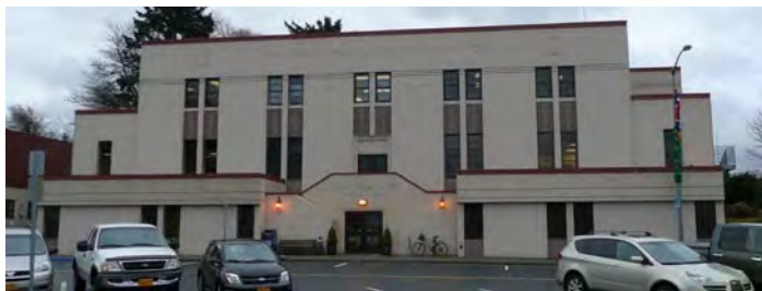
Figure 5. Example of Modernistic, Art Deco style building, 100 East Lincoln Street (©TNSDS 2014). The Sitka U.S. Post Office and Court House is listed on the NRHP for its association with 1930s and 1940s government activities in Sitka, and for being exemplary of the Modernistic Movement in federal architecture. It was designed by Gilbert Stanley Underwood, a prominent architect who designed numerous federal buildings across the U.S., including the Anchorage Federal Building. 23
