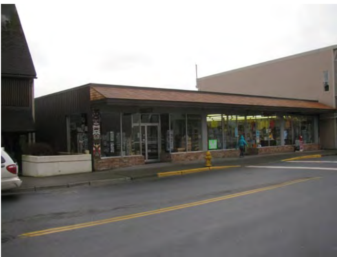
Figure 28. The Ben Franklin Store, 214 Lincoln Street, view facing southwest (©TNSDS 2014).
