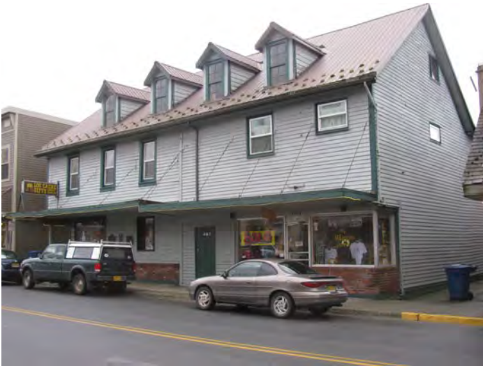
Figure 3. Example of a Russian Colonial style building, 206 East Lincoln Street (©TNSDS 2014). Also known as the Tilson Building (Building 29), this example of Russian Colonial architecture has compromised architectural significance due to alterations; the building was originally a log structure, with wood shingle roof, and has seen numerous changes through time. It is currently a National Historic Landmark, listed for its association with U.S. Political and Military Affairs. 17
