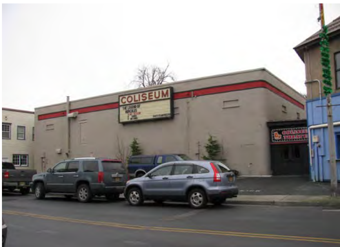
Figure 45. The Coliseum Theater / Moose Lanes, 331 Lincoln Street, view facing west (©TNSDS 2014).
