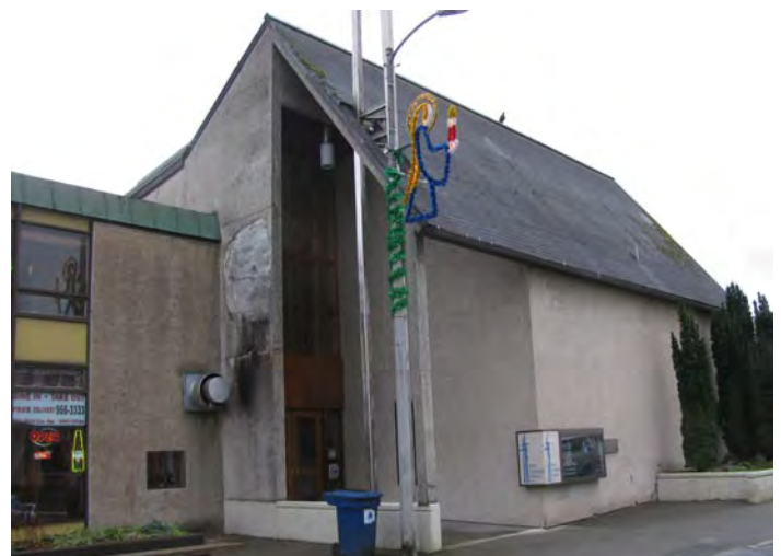
Figure 29. The Sitka Lutheran Church, 224 Lincoln Street, view facing southwest (©TNSDS 2014).
