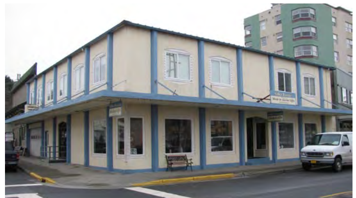
Figure 40. Sitka Bazaar, 215 Lincoln Street, view facing north (©TNSDS 2014).
