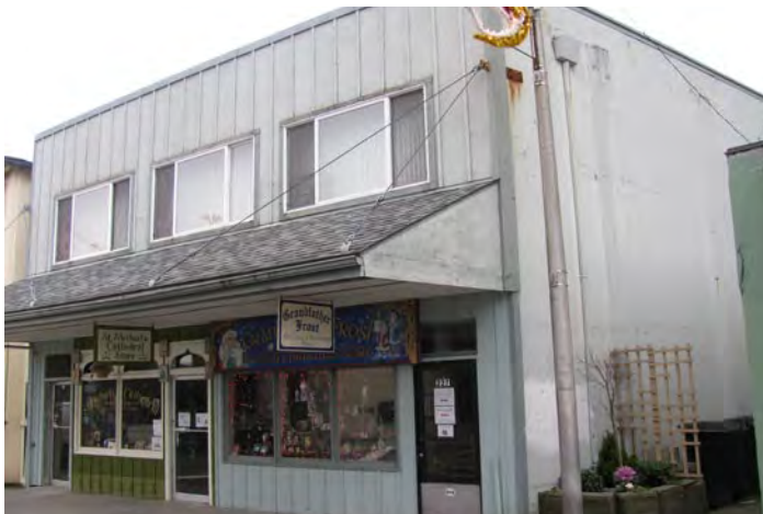
Figure 41. Saint Michael's Store, 221 Lincoln Street, view facing west (©TNSDS 2014).
