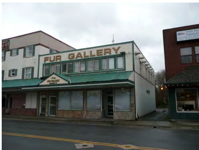
Figure 20. The Fur Gallery, 108 Lincoln Street, view facing south-south-east (©TNSDS 2014).
