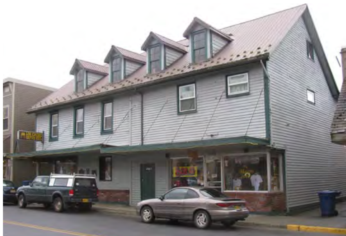
Figure 26. The Tilson Building/Russian American Building Number 29 at 206 Lincoln Street, view facing southeast (©TNSDS 2014).
